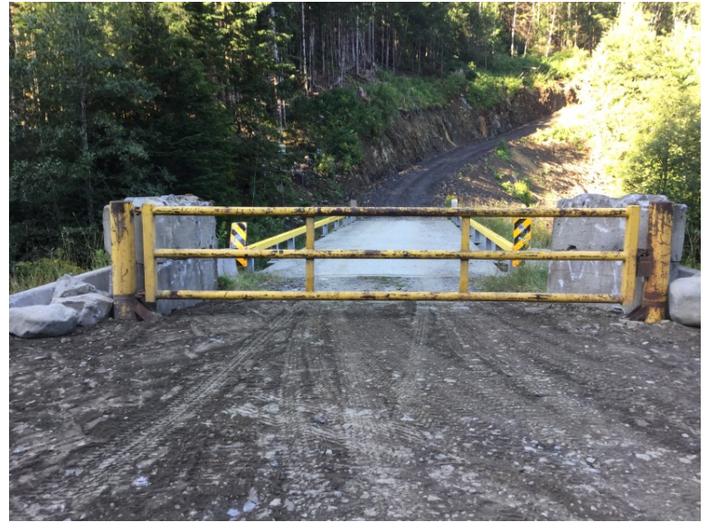
Approach from Right Bank when facing downstream
