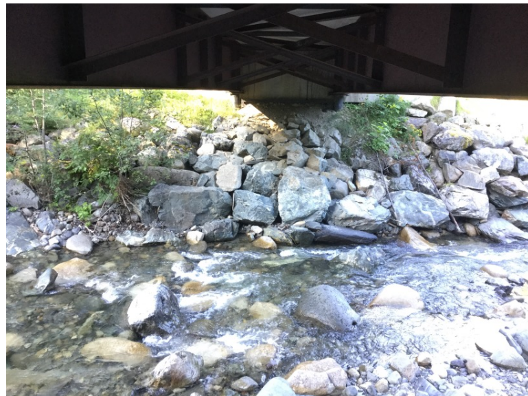
Left Bank Abutment when facing downstream
