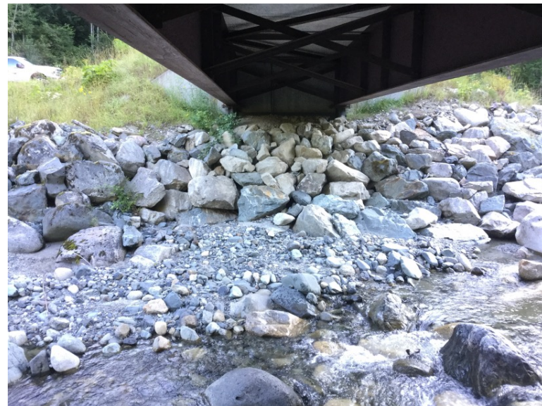
Right Bank Abutment when facing downstream
